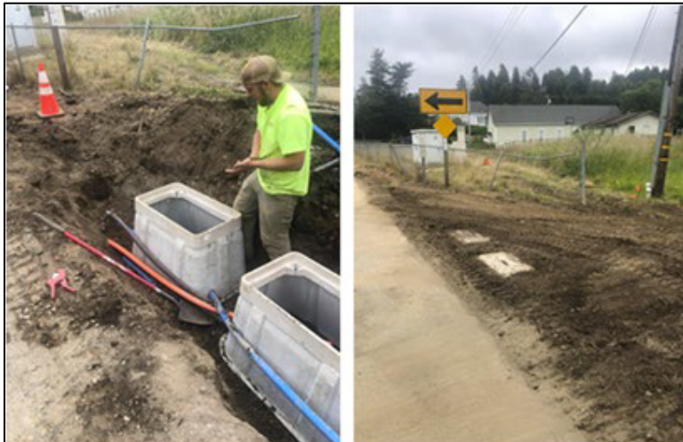
Photograph 7. Vault Construction Before and After
