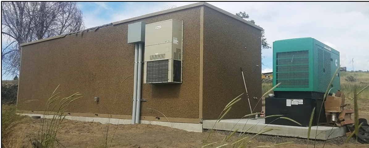
Photograph 6. Typical In-Line Amplifier
