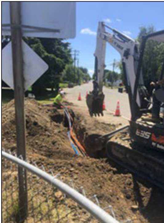
Photograph 1. Trenching Example
