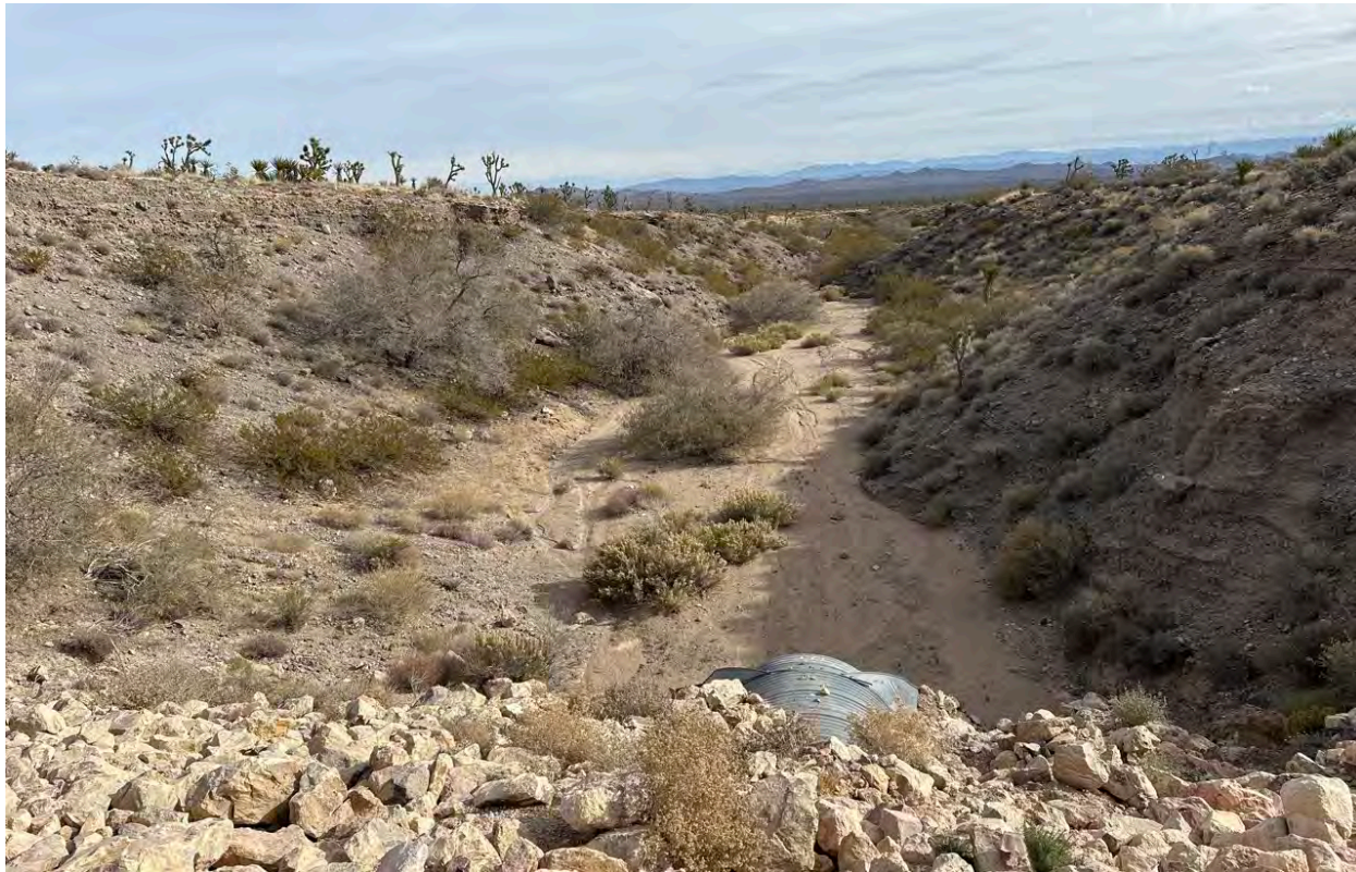
Photograph 5: Representative photo of a confined desert wash as seen from the top of Walking Box Ranch Road facing east. Note the large culvert which conveys flows under the roadway.
