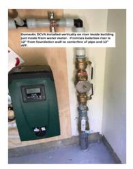
The double check valve assembly (DC) is commonly used to protect against backflow hazards that do not pose a health risk. They may be used under continuous pressure and protect against both backsiphonage and backpressure conditions.
