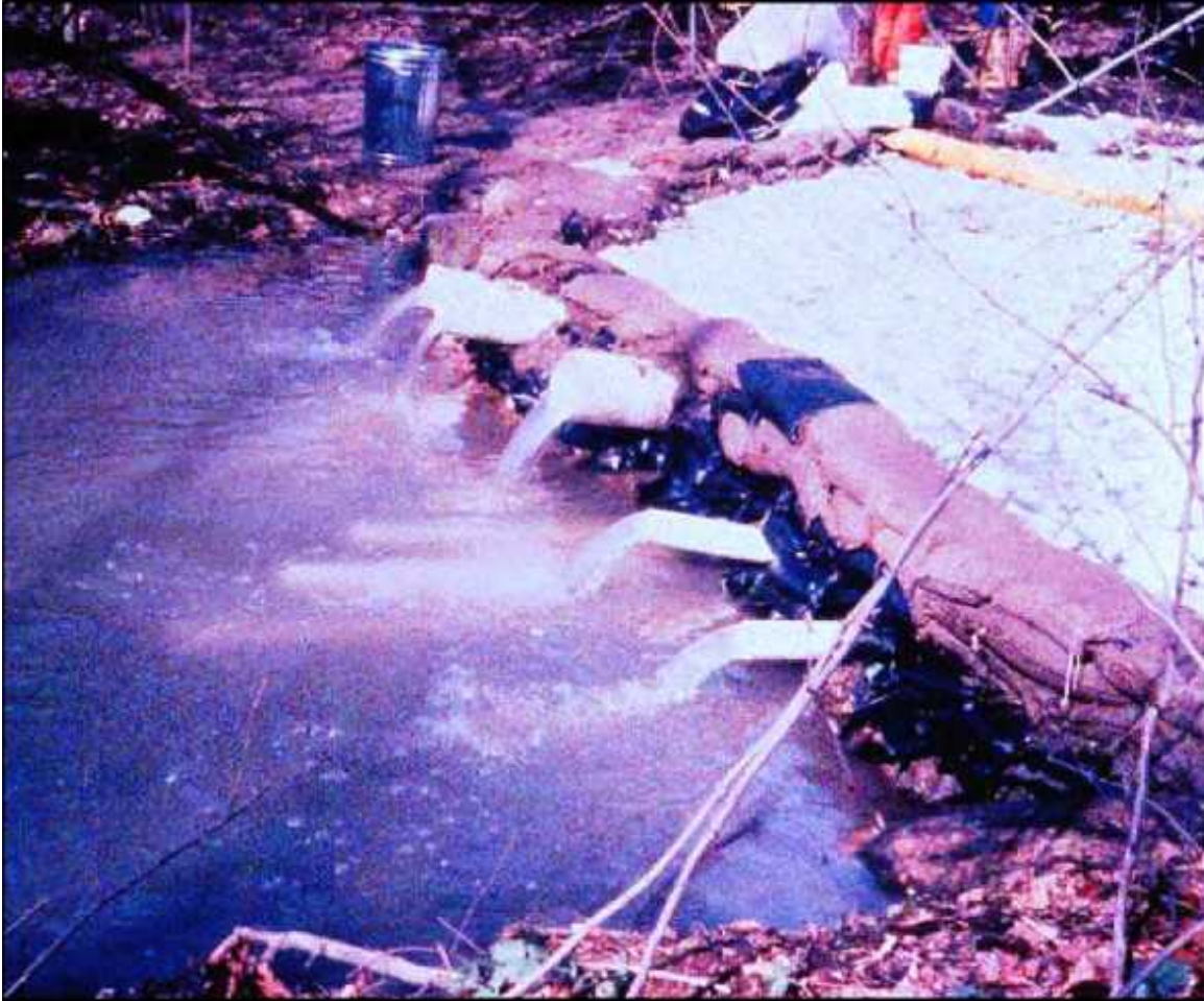
Sandbag underflow dam
