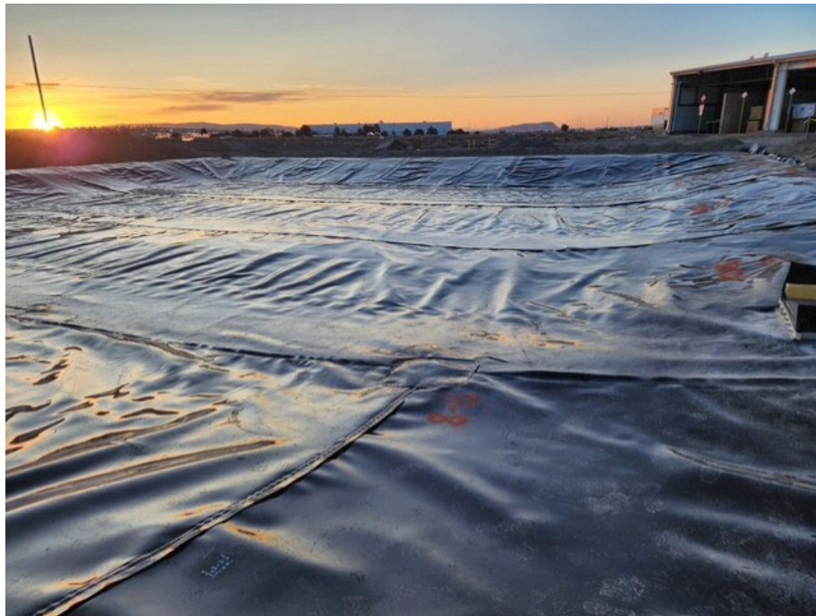
Photo 22 –Completed liner for stormwater pond 06/24/25.
