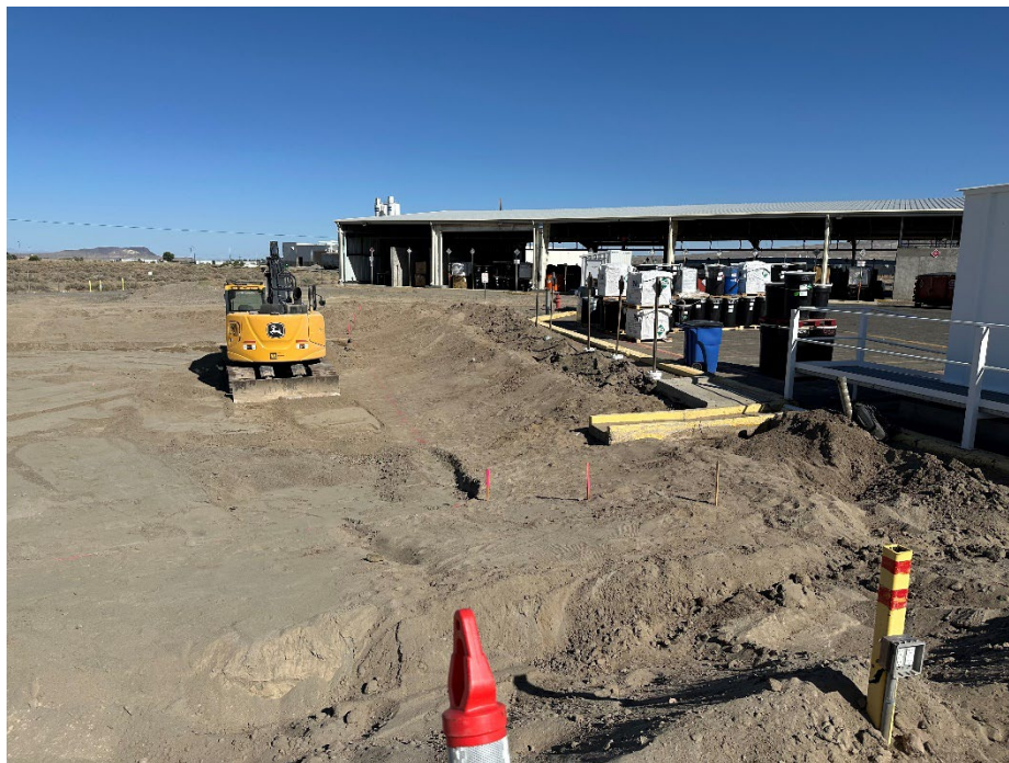
Photo 10 – Stormwater pond after old liner removal 6/17/25. Facing southeast.
