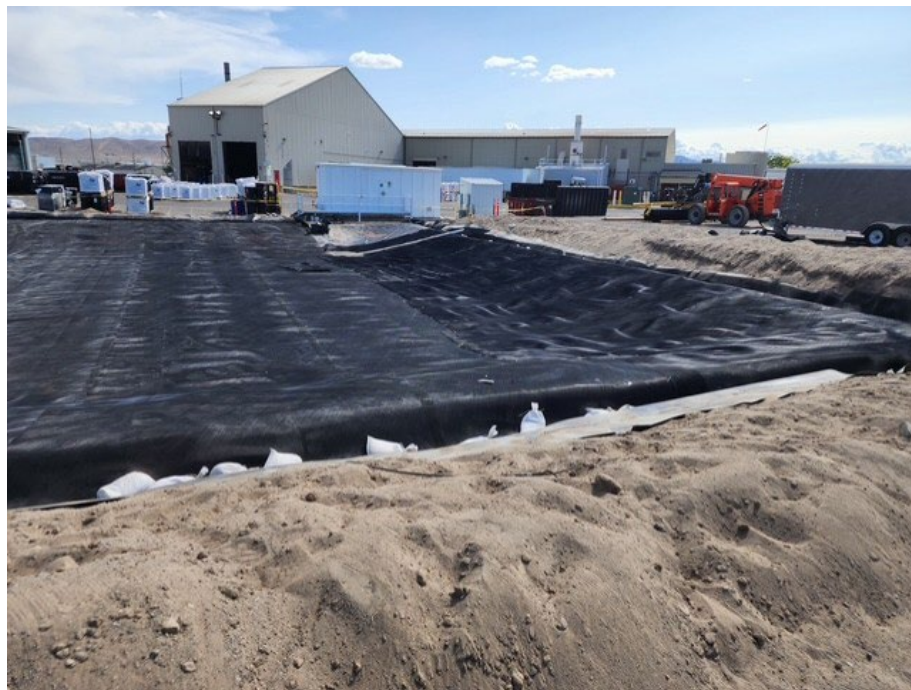
Photo 18 – Stormwater pond trenching for anchoring of liners.
