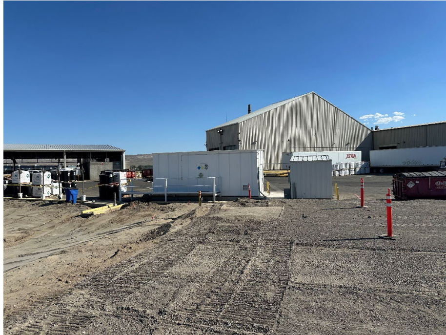
Photo 13 – Stormwater pond grading 6/18/25.
