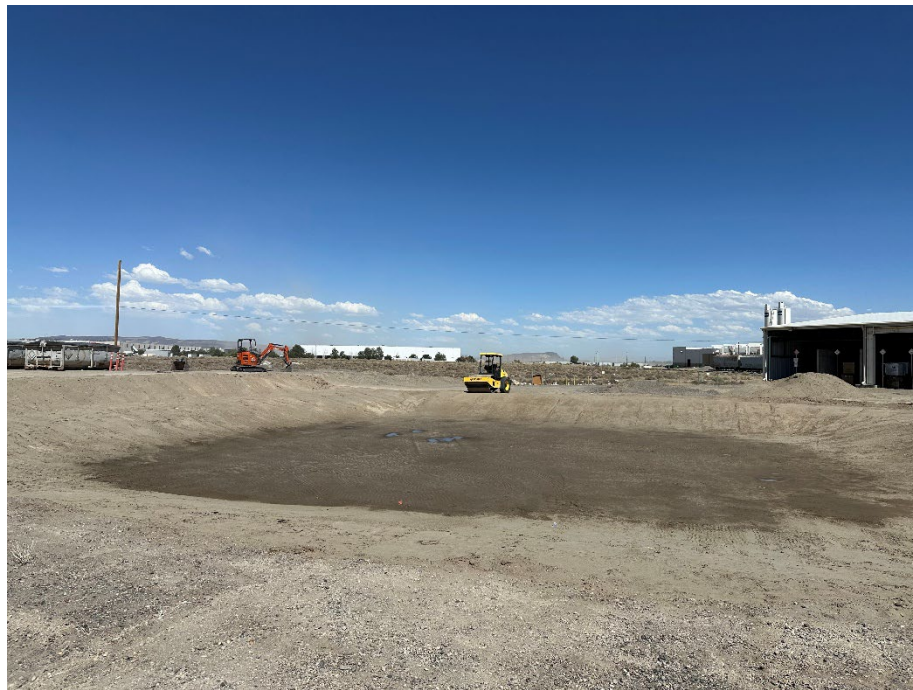
Photo 14 – Stormwater pond wetting of sand for compaction testing 6/19/25.
