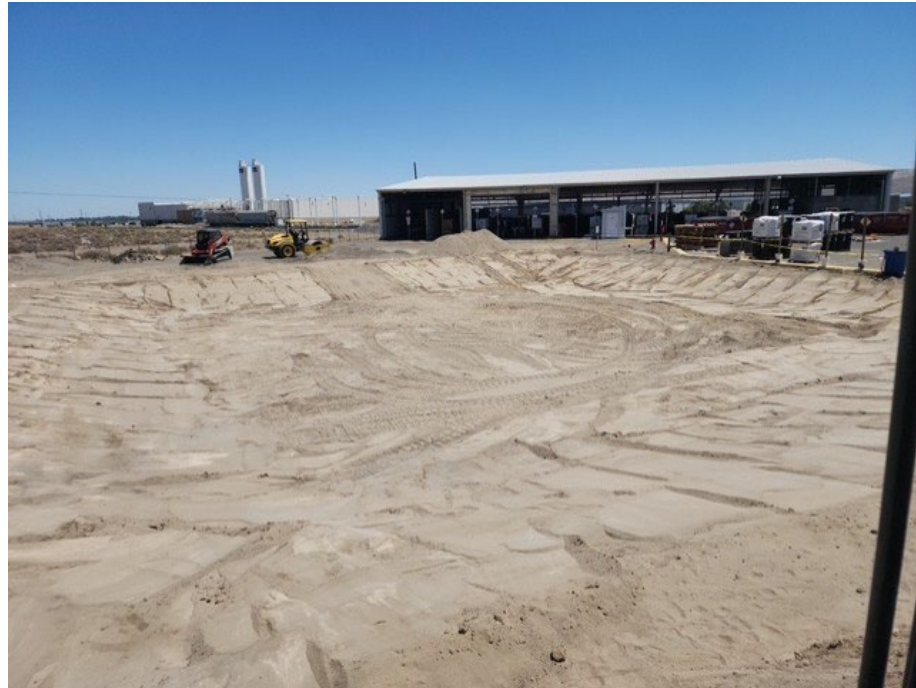
Photo 15 — Stormwater pond grading prior to trenching for liner anchoring. Facing south towards the East Container Storage Building.
