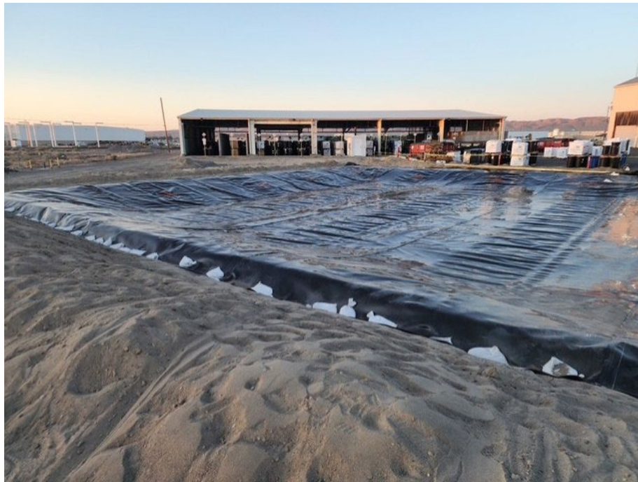
Photo 20 – Stormwater pond trenching for anchoring of liners. Facing south towards the East Container Storage Building.
