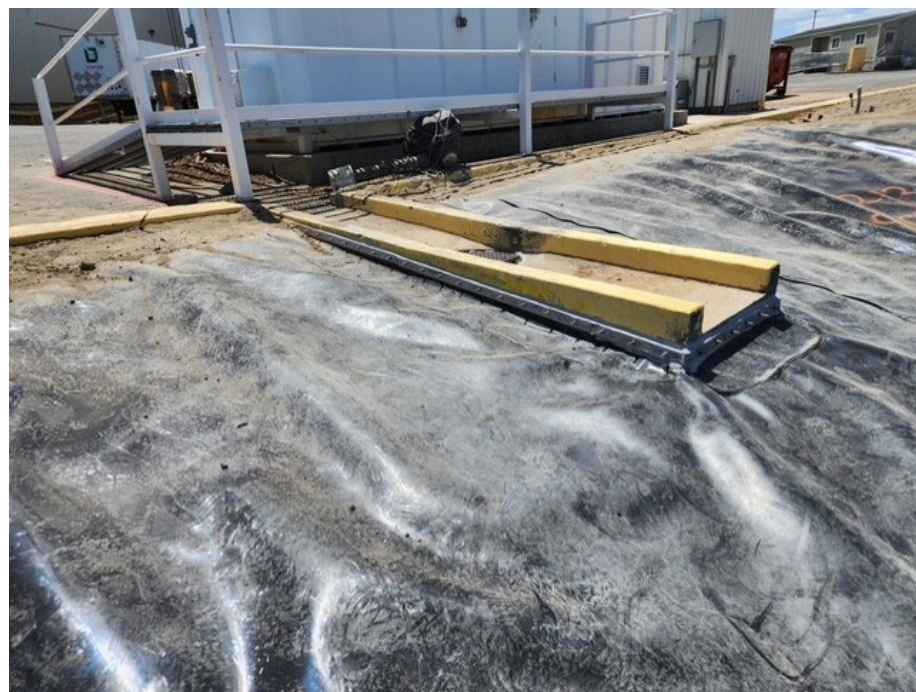
Photo 26 – Completed stormwater pond spillway 06/25/25.
