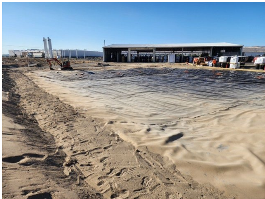
Photo 24 – Completed stormwater pond 06/25/25.
