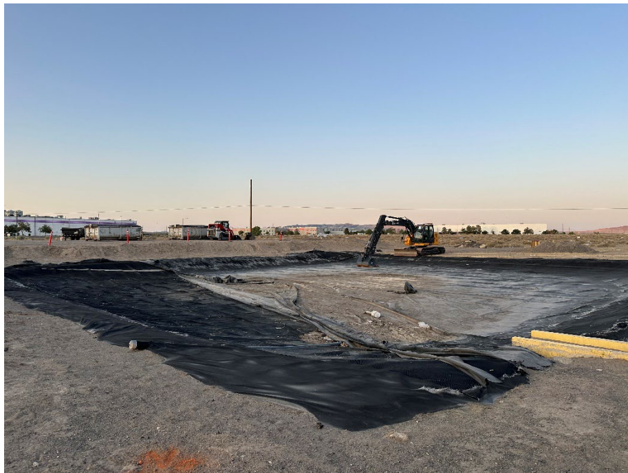
Photo 8 – Stormwater removal of primary liner 06/16/25.
