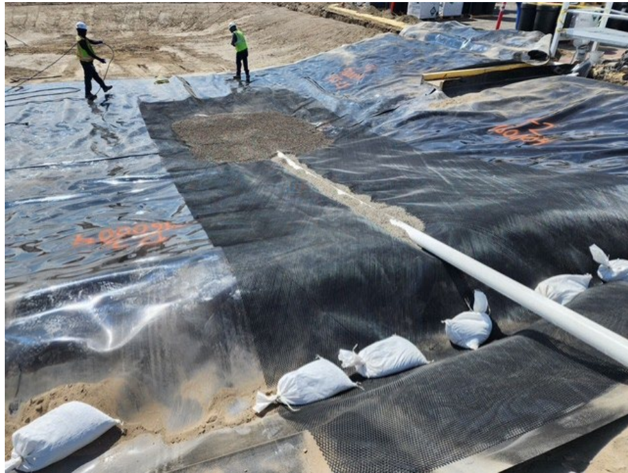
Photo 17 – Stormwater pond leak detection piping (4 inch diameter schedule 40 PVC with 10 feet of 0.020 slot screen bedded in pea gravel) prior to covering with primary liner.
