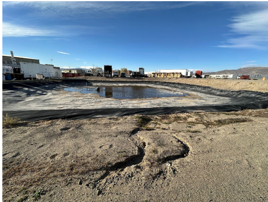
Photo 2 – Stormwater pond pre-construction 11/11/24.
