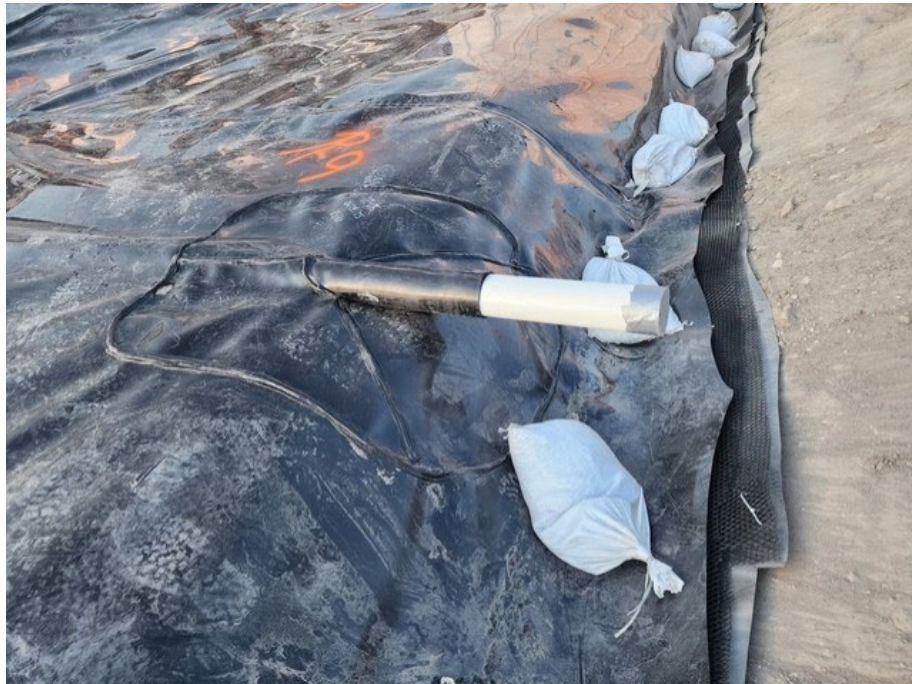
Photo 19 – Stormwater pond leak detection piping prior to anchoring of liners. West corner of pond.
