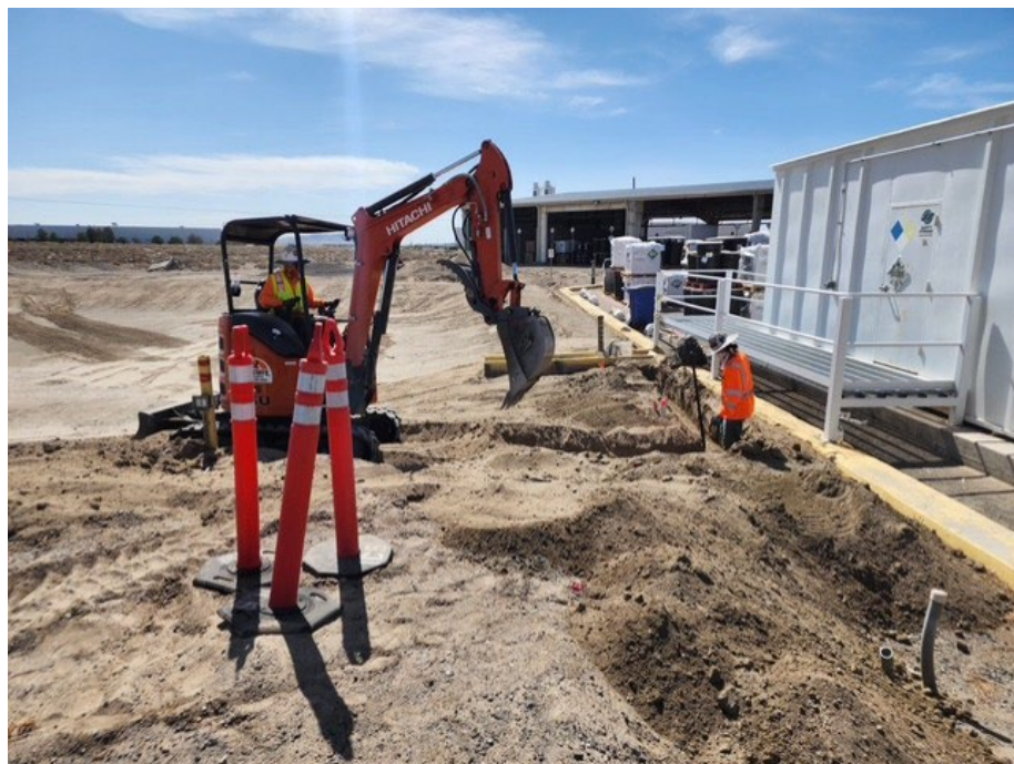
Photo 16 – Stormwater pond trenching for liner anchoring. Facing southeast.
