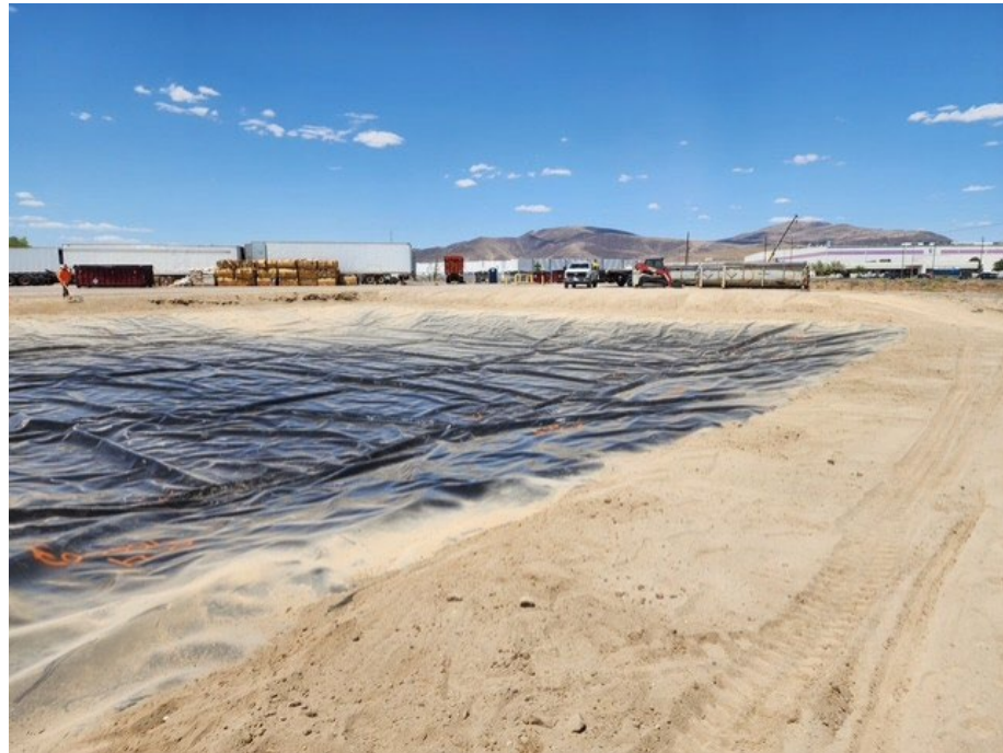
Photo 23 – Completed stormwater pond 06/25/25.
