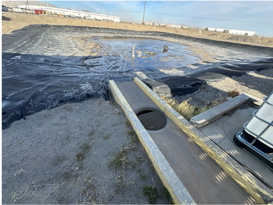
Photo 5 – Stormwater pond spillway 11/11/24.
