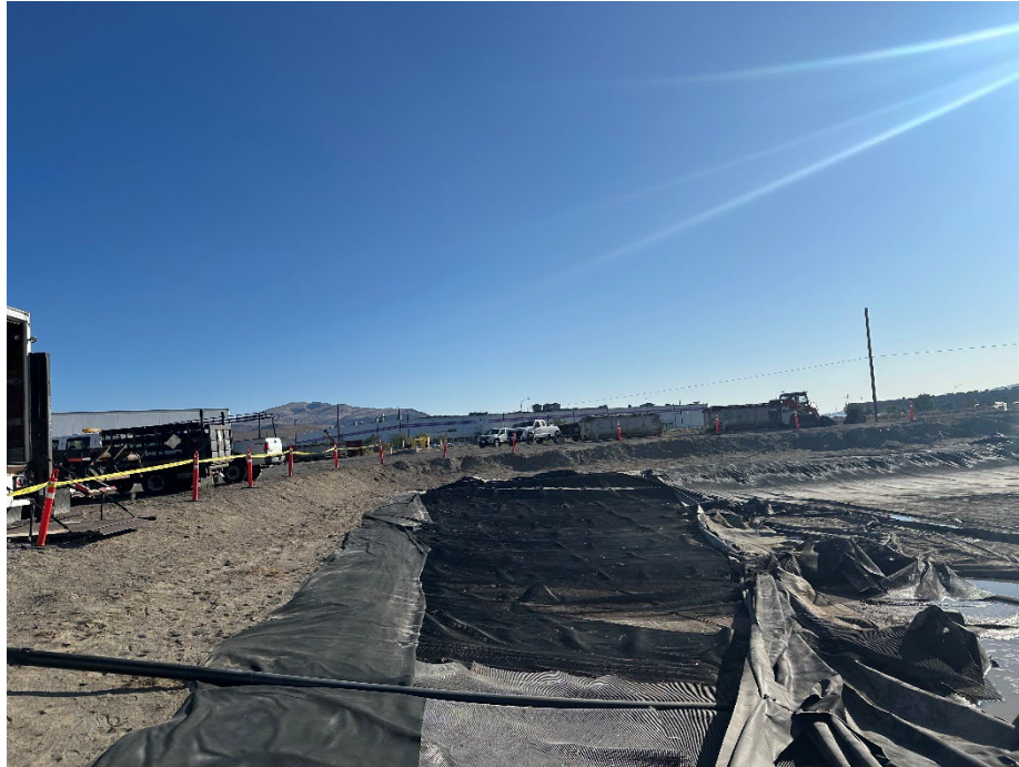
Photo 7 – Stormwater removal of primary liner 6/17/25
