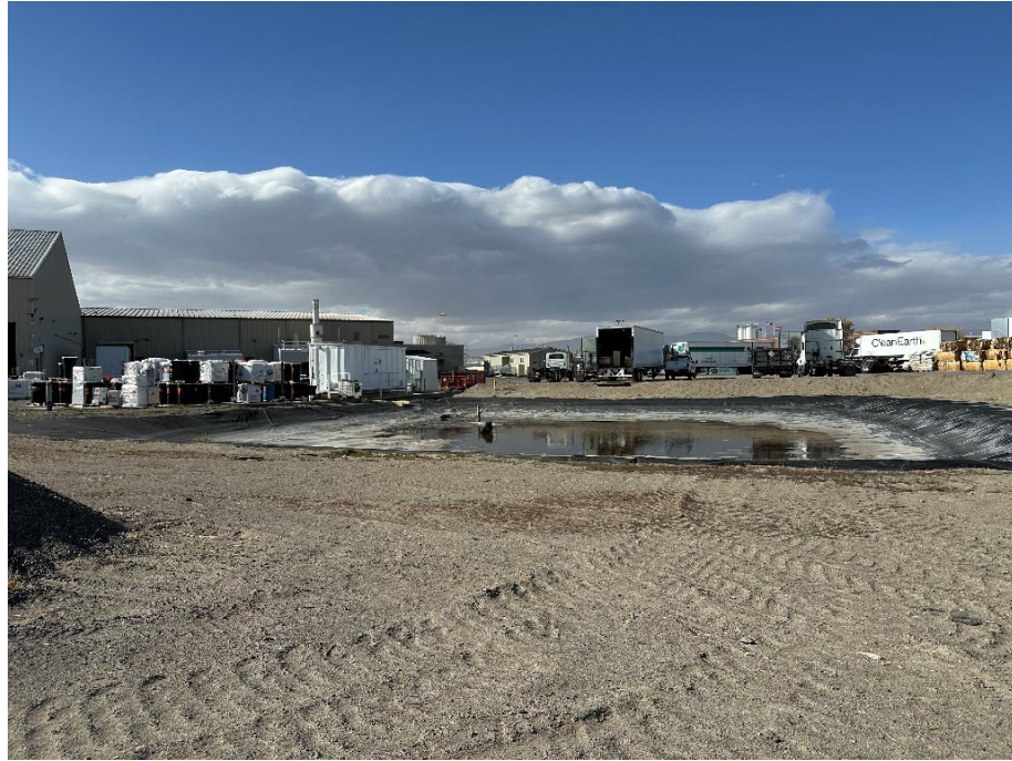
Photo 1 – Stormwater pond pre-construction 11/11/24.
