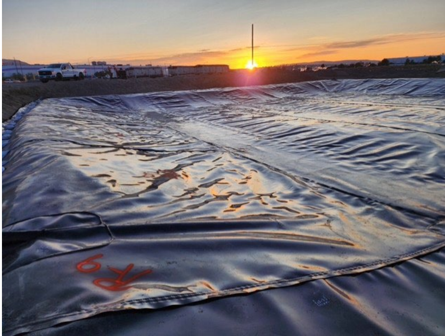
Photo 21 – Completed liner for stormwater pond 06/24/25.
