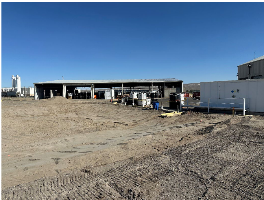
Photo 12 – Stormwater pond grading 6/18/25
