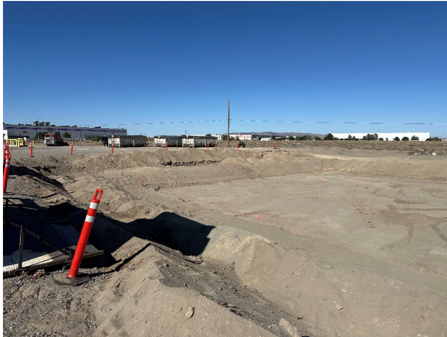
Photo 9 – Stormwater pond after old liner removal 6/17/25 Facing north.
