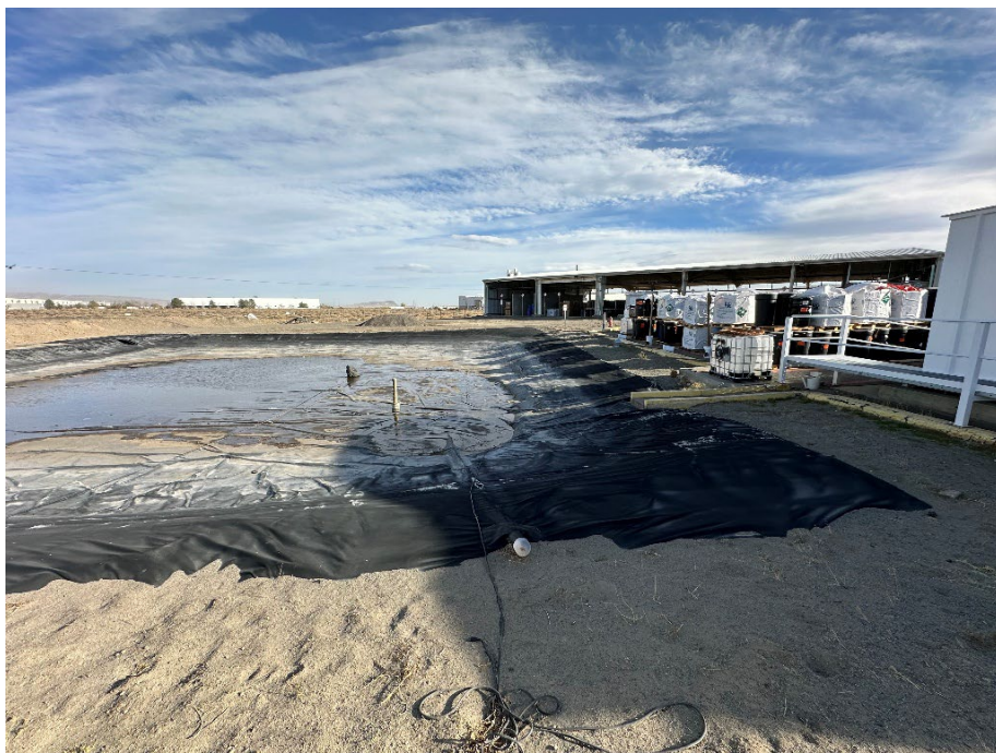
Photo 4 – Stormwater pond pre-construction 11/11/24.
