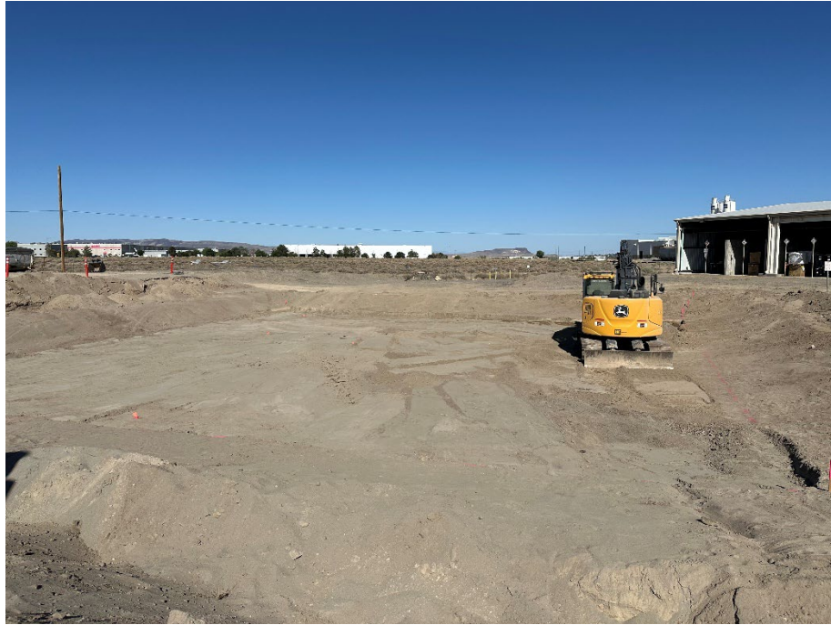
Photo 11 – Stormwater pond grading 6/18/25
