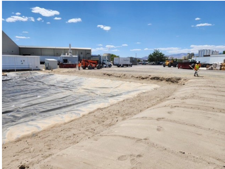
Photo 25 – Completed stormwater pond 06/25/25.
