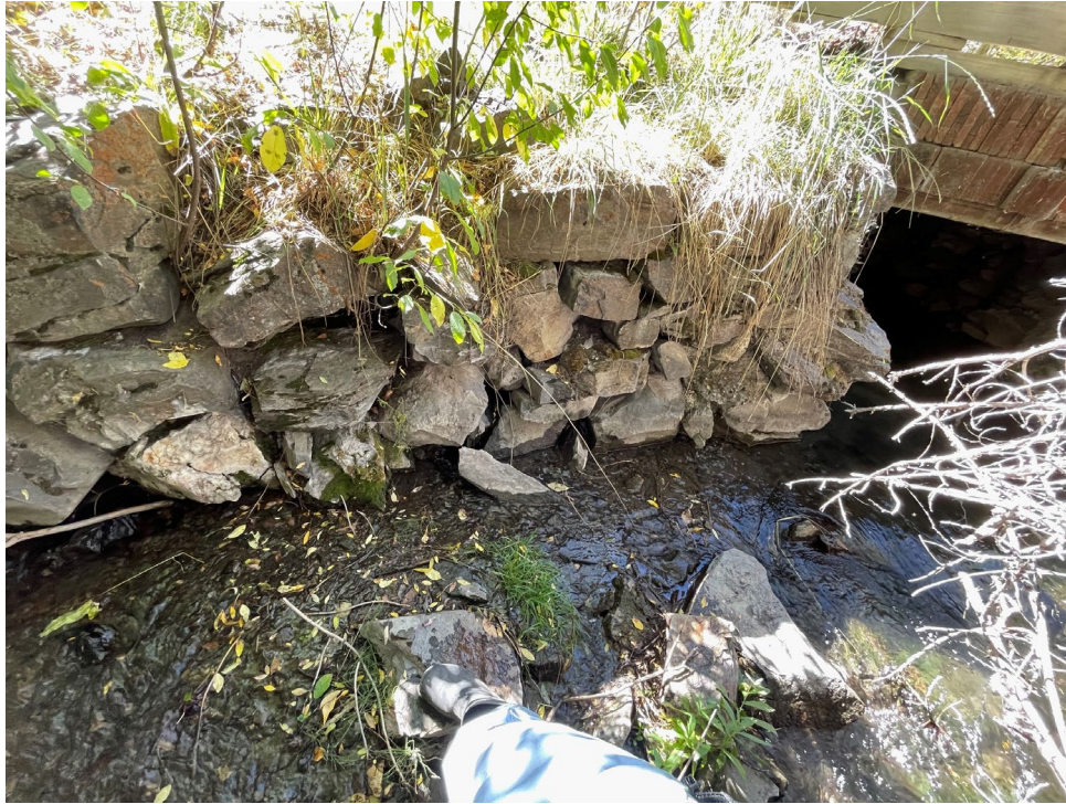
Flow through A1 wingwall downstream
