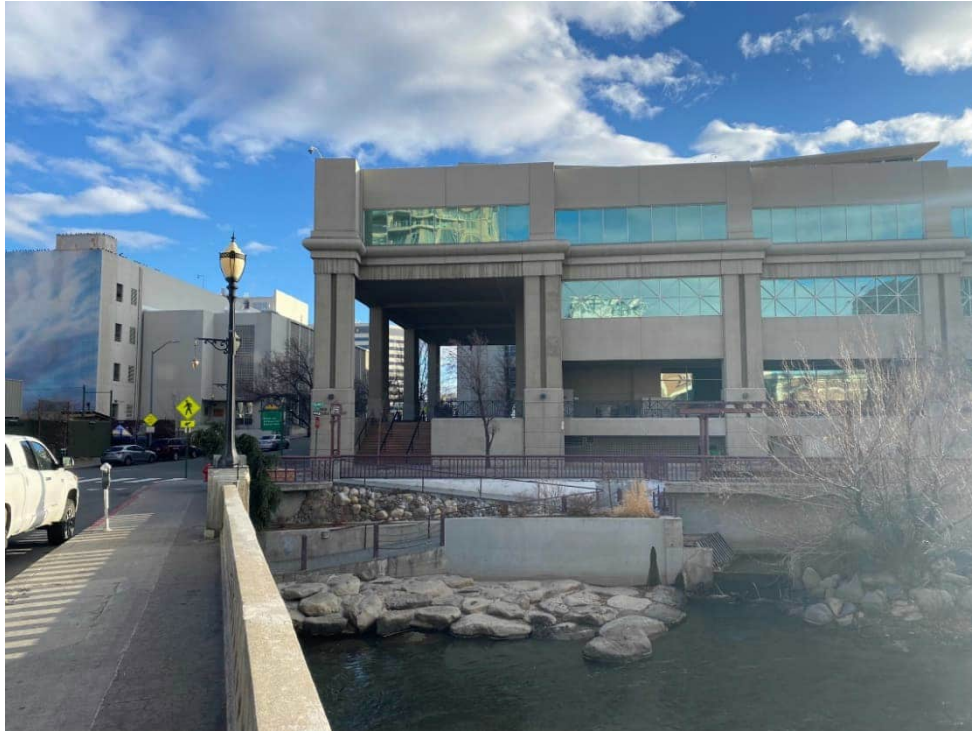
Facing south toward the existing river access ramp, grouted riprap structure, and Cochrane Ditch inlet structure from the western side of the Sierra Street Bridge.
