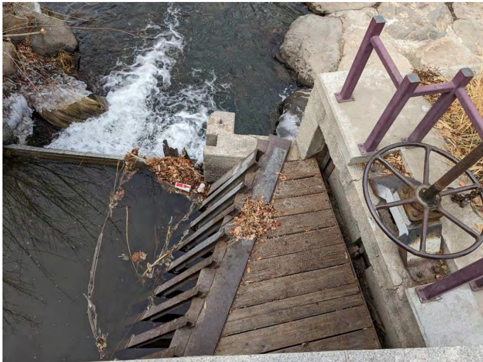
Looking down at the existing Cochrane Ditch inlet structure.
