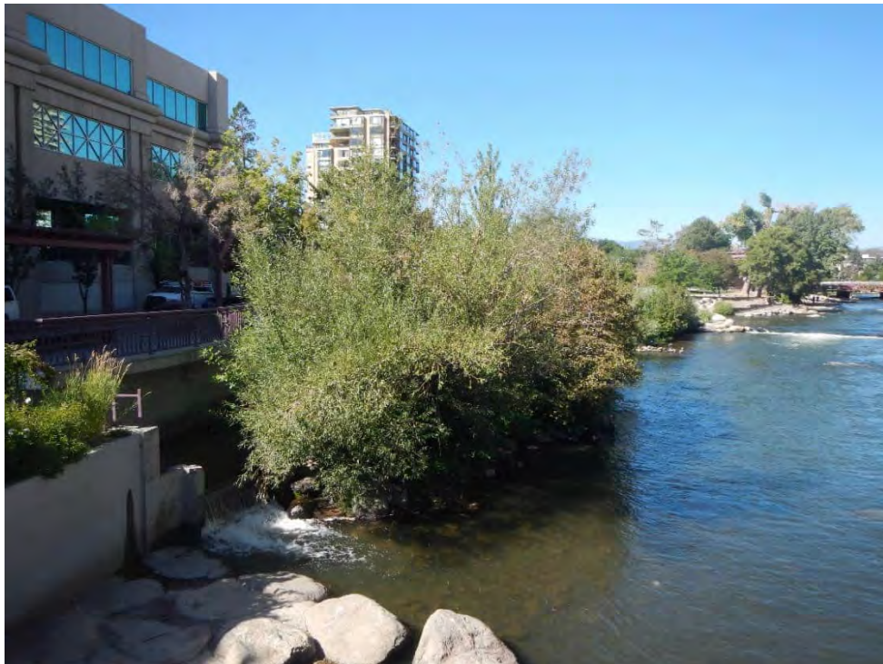
Looking upstream toward the Cochrane Ditch inlet and gravel bar wetland from the existing ramp and grouted riprap along the southern side of the river.
