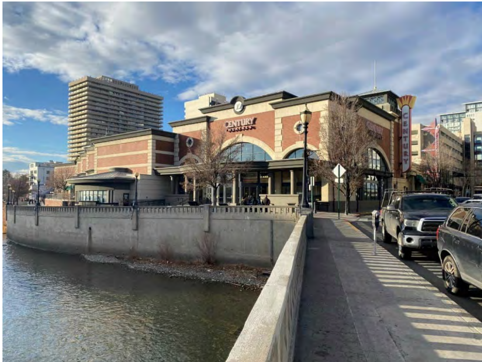
Looking north toward the northern floodwall from the western side of the Sierra Street Bridge.
