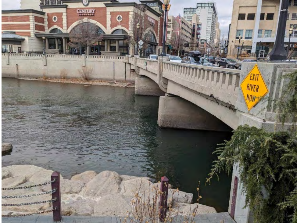
Facing north across the river from the existing river access ramp.
