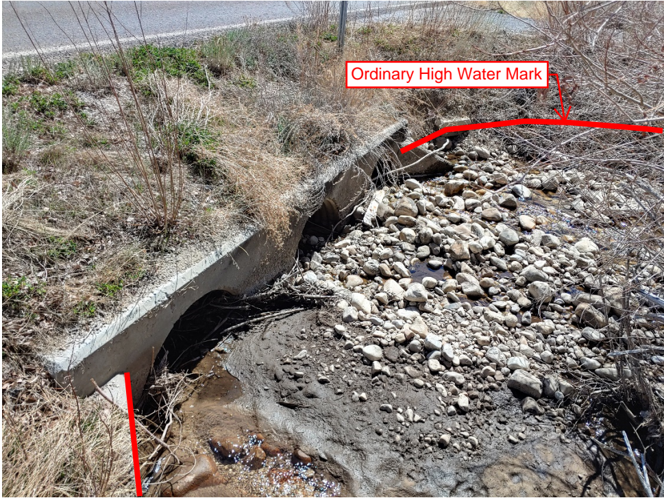
Lehman Creek / SR-487 Culvert Crossing (Upstream, looking south)
