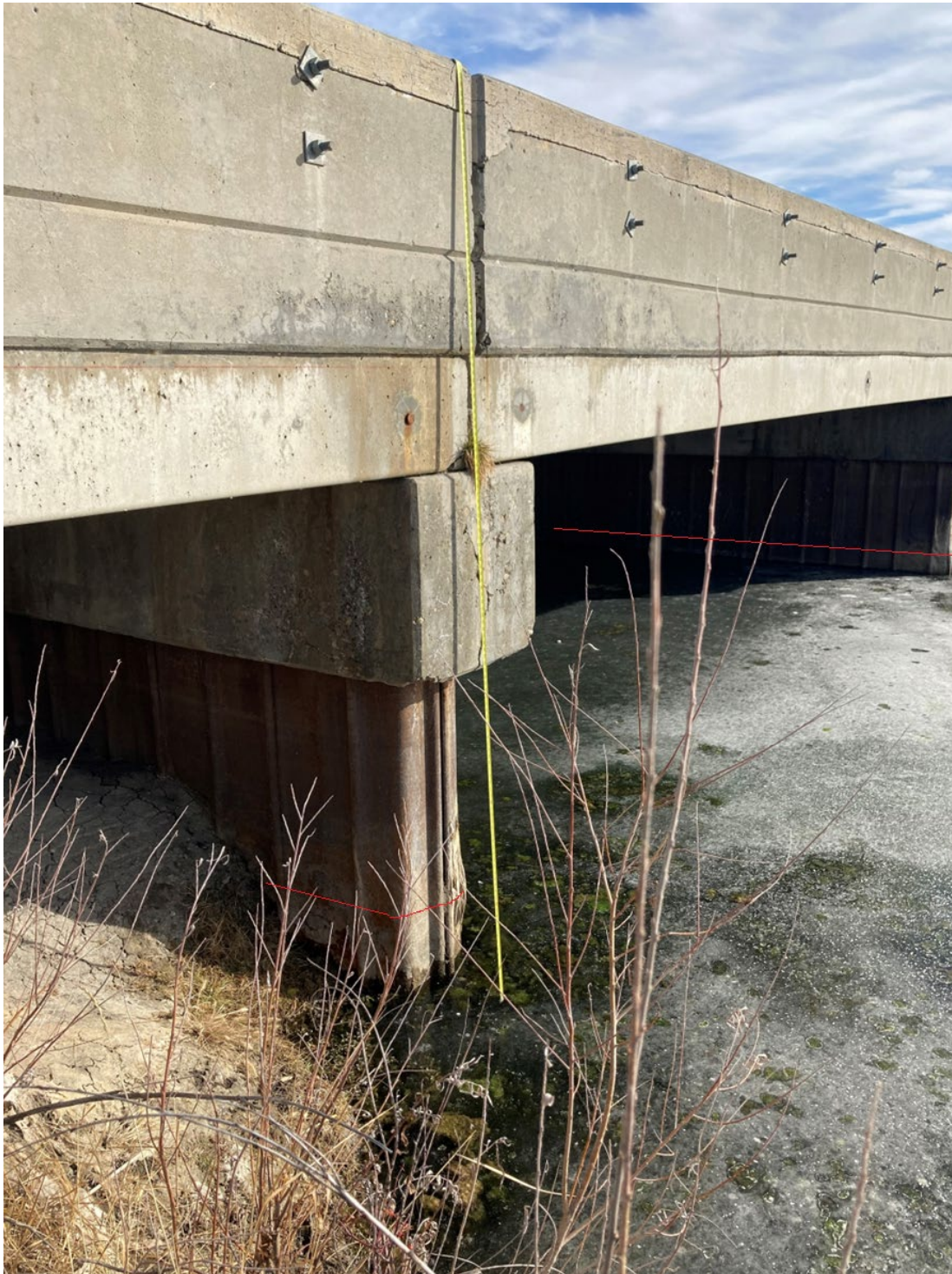
EL 1.35 B-3340 (Downstream, Looking Upstream to the Northeast)
