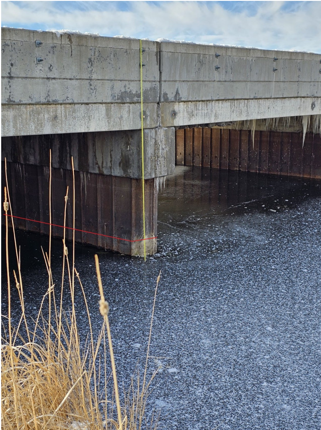
EL 1.35 B-3340 (Upstream, Looking Downstream to the Southwest)
