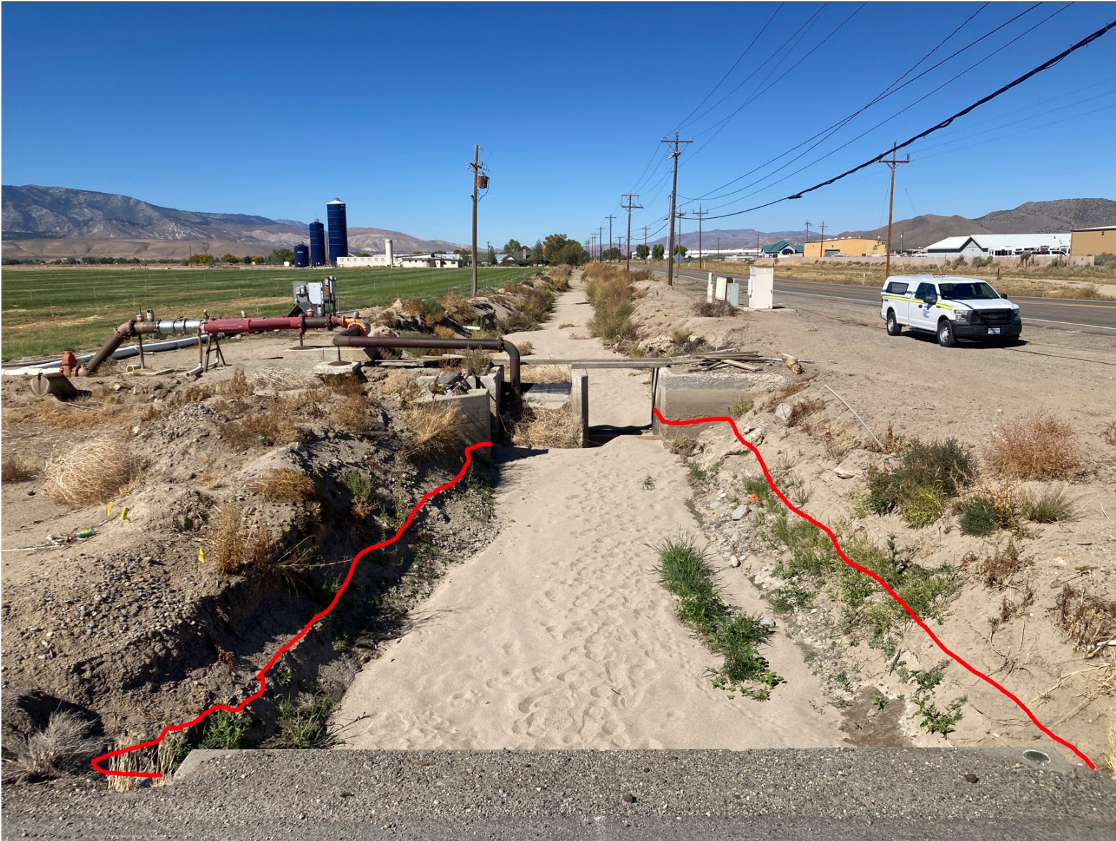
Photopoint 4 – Heybourne Ditch outlet looking North (downstream).
