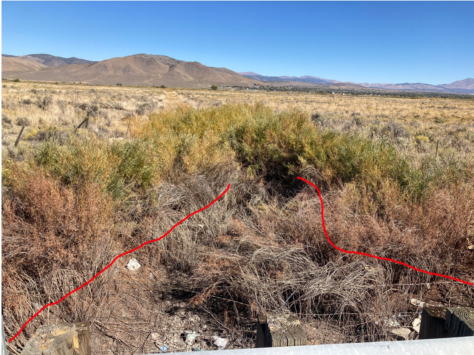
Photopoint 2 – DO 30.374 Outlet looking East (downstream).
