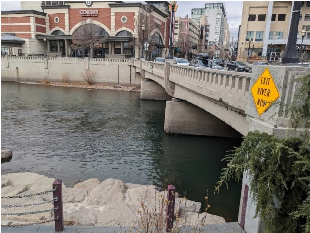
Photo 5: Facing north from the southwest bridge corner at the existing river access ramp.
