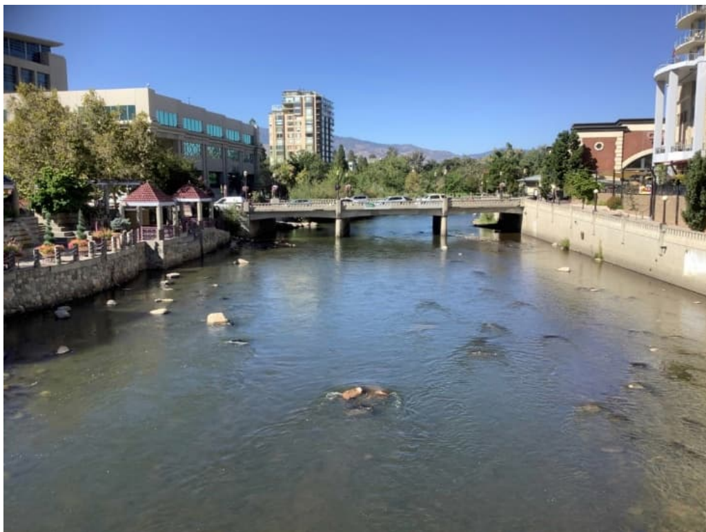
Photo 1: Facing upstream toward the Sierra Street bridge from Virginia Street.
