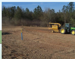
Reseeding the right-of-way
