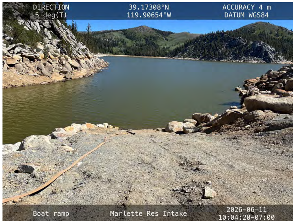
Photo 3. Existing access route to be used to launch barge that is needed to hoist and raise/lower the old and new intake structure for removal/installation. If needed, approximately 420 CY of rock will be placed to reduce slope, resulting in 1,732 SF (0.04 ac) of permanent impact.
