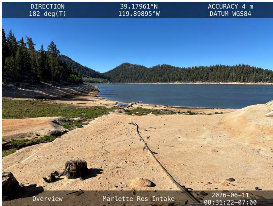
Photo 1. Photo taken from normal water edge looking south along water line extending into drained lake. Water intake structure is located approximately 300 feet lakeward below water. Approximately 64 SF / impact to AR-1: Marlette Lake
