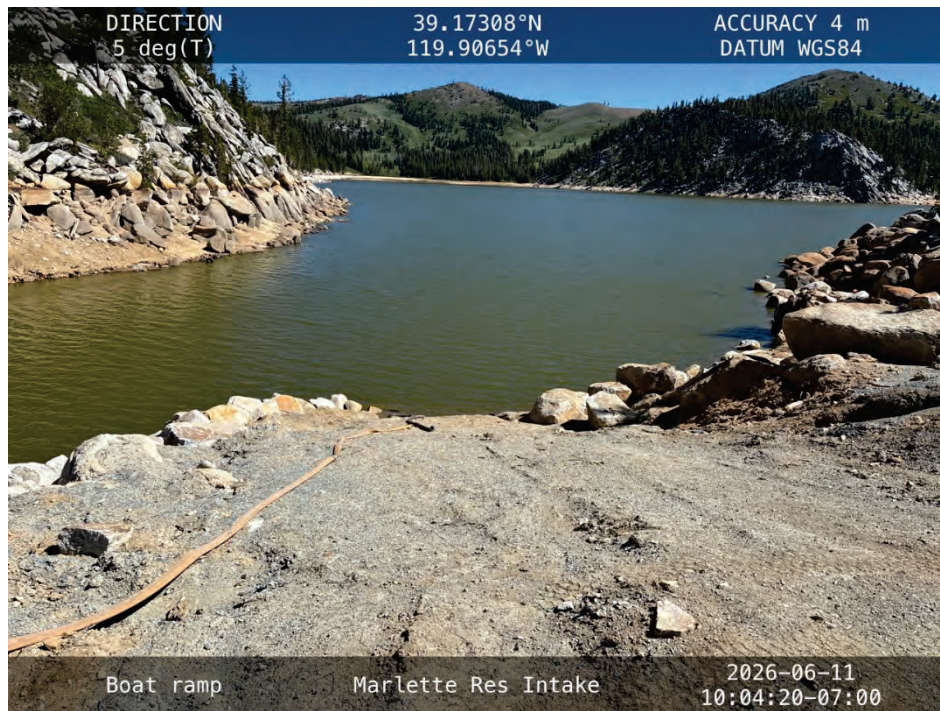
Photo 5. Existing boat ramp to be used to launch barge that is needed to hoist and raise/lower the old and new intake structure for removal/installation.
