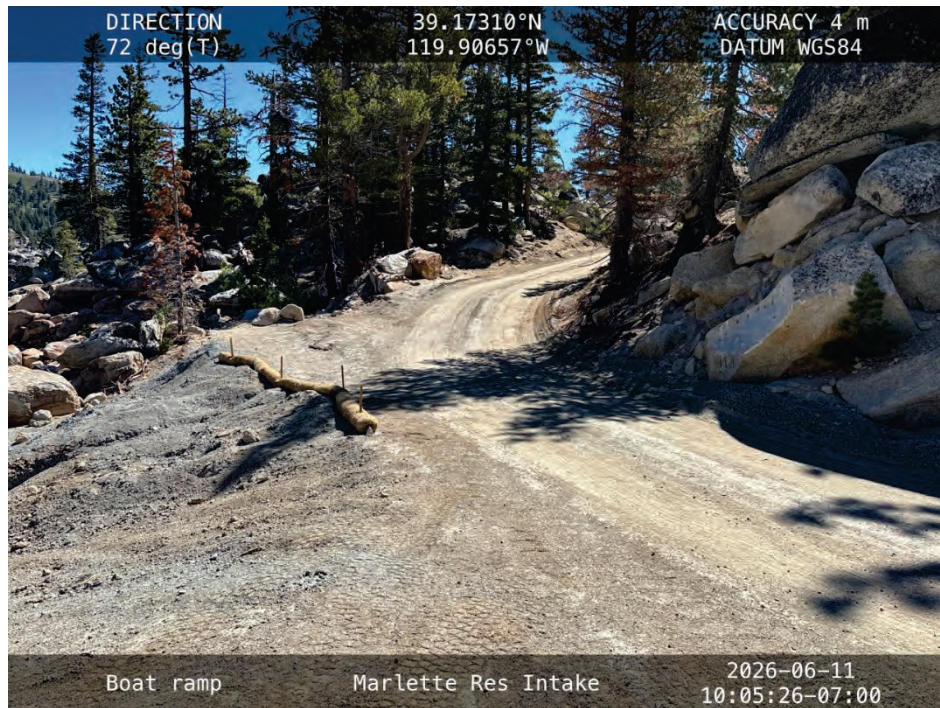
Photo 6. Existing access road to boat ramp.
