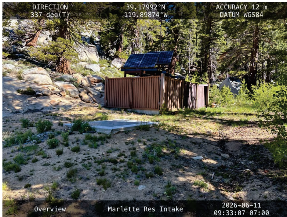
Photo 3. View of existing pump house and adjacent upland vegetation
