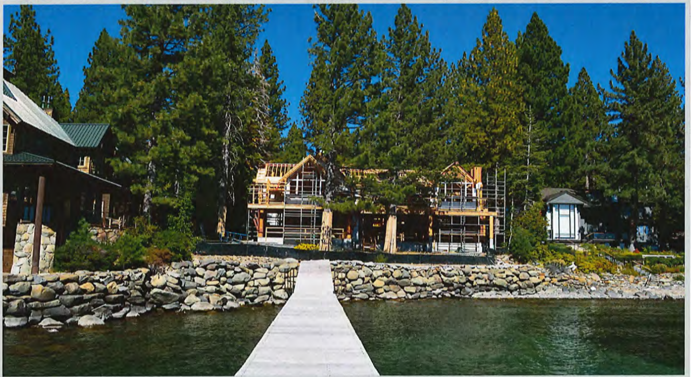
VIEWING NORTHERLY FROM SUBJECT PIER STRUCTURE
