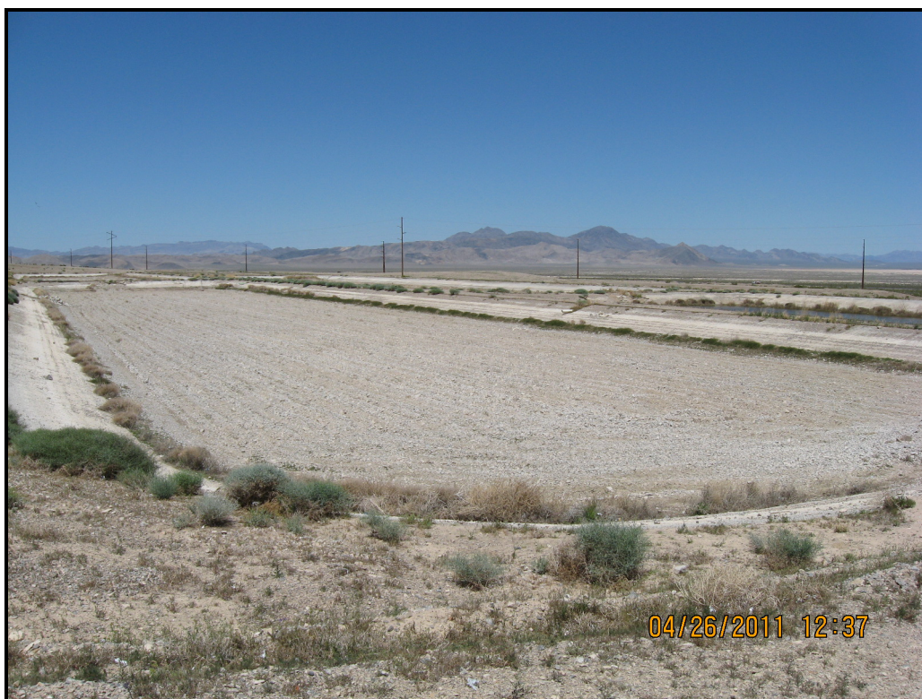
Figure 1. An Example of a Dry RIB in Southern Nevada
