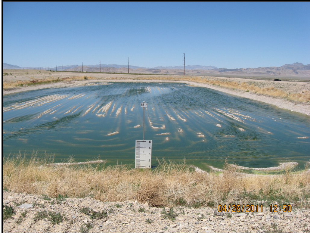
Figure 2. An RIB that Shows Treated Effluent Percolating into the Subsurface
