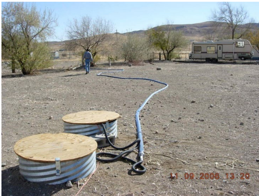
Fig. 2 – Example (unauthorized bypass of effluent)
