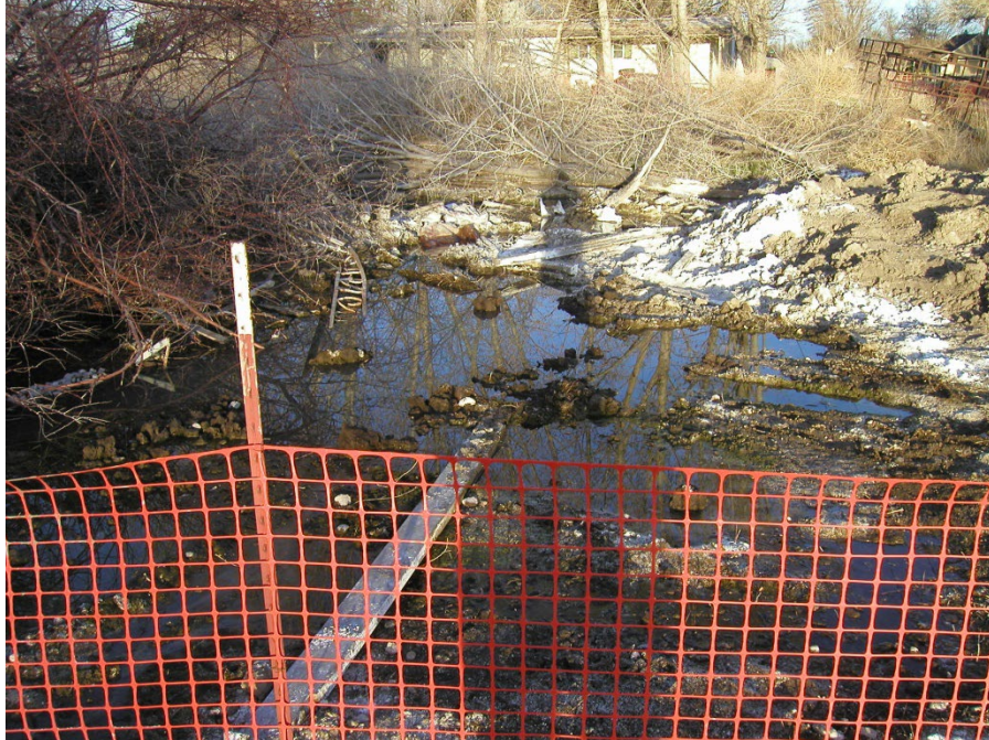
Fig. 1 – Example (failed leach field)
