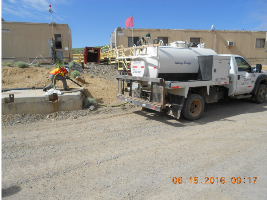
Fig. 4 - Pumping a Vault Holding Tank
