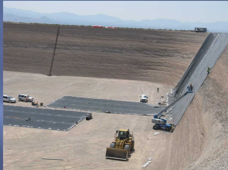
Modern waste cell (ca. post-1992)
