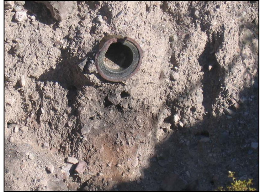
Photo 22 – Exposed pipeline, NE of mill site. January 9, 2007.
