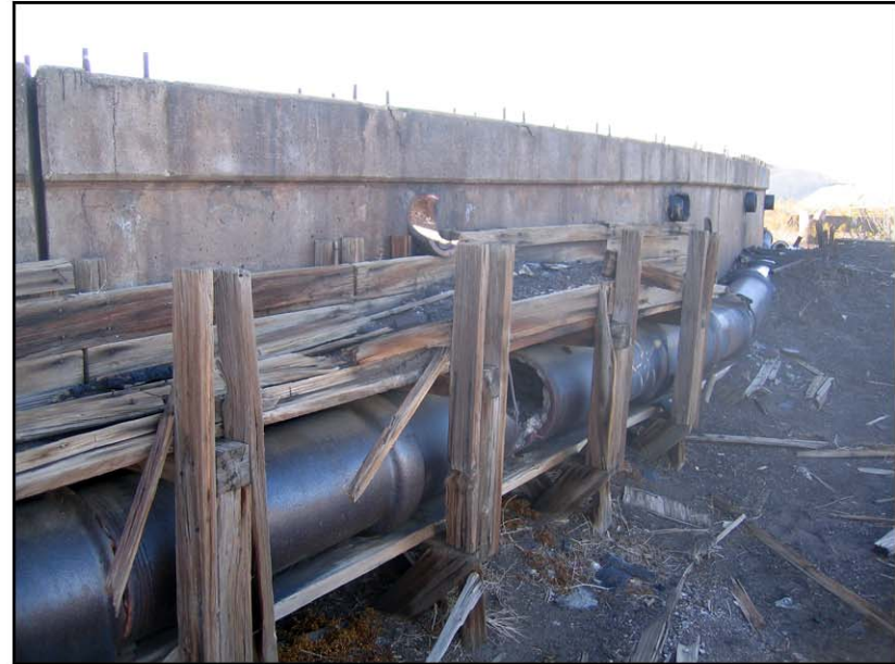
Photo 18 – Thickener showing vitrified clay pipe with residues. January 9, 2007.
