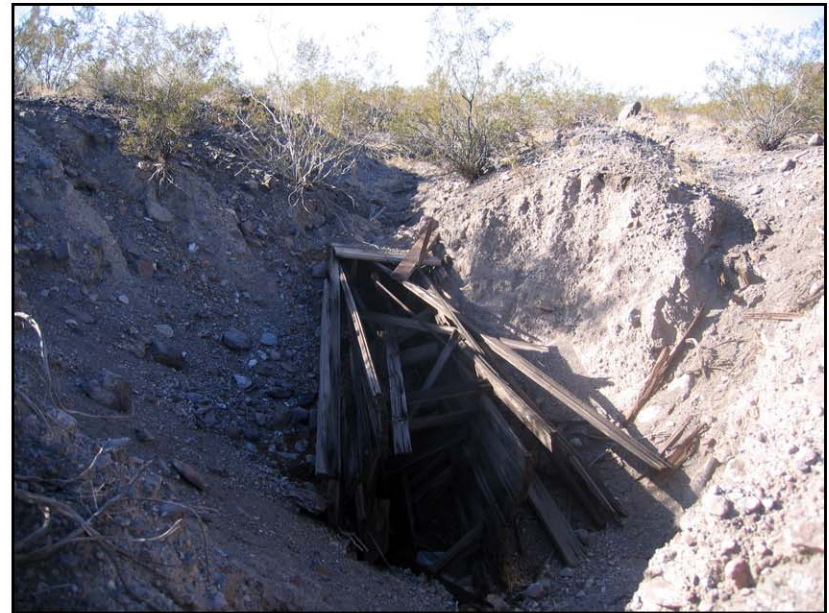
Photo 24 – Remains of subsurface wooden drainage, NE of mill site, facing W. January 9, 2007.
