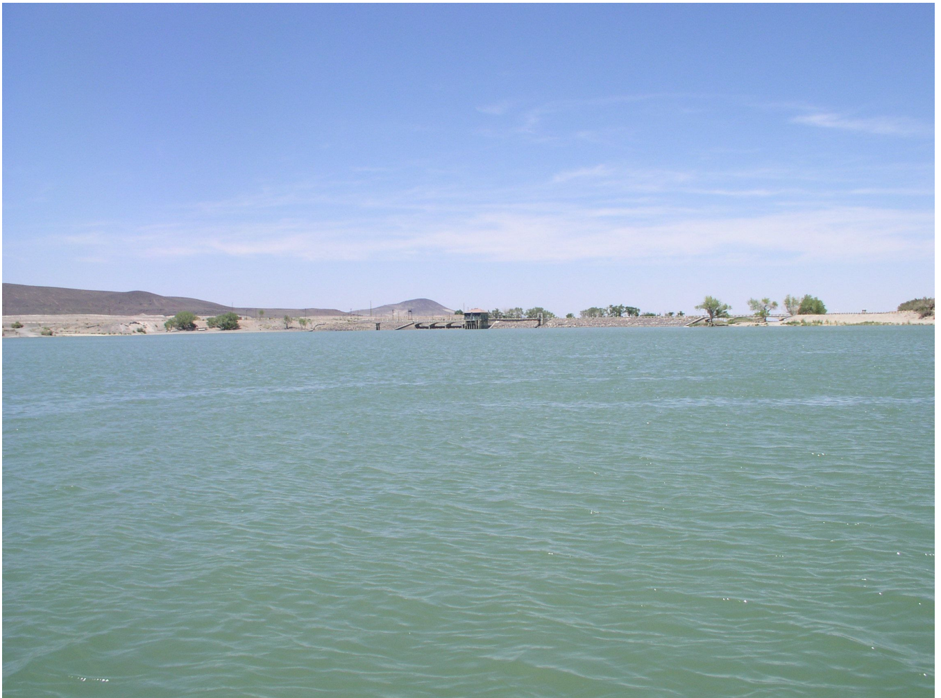
Near Dam Site LR5
