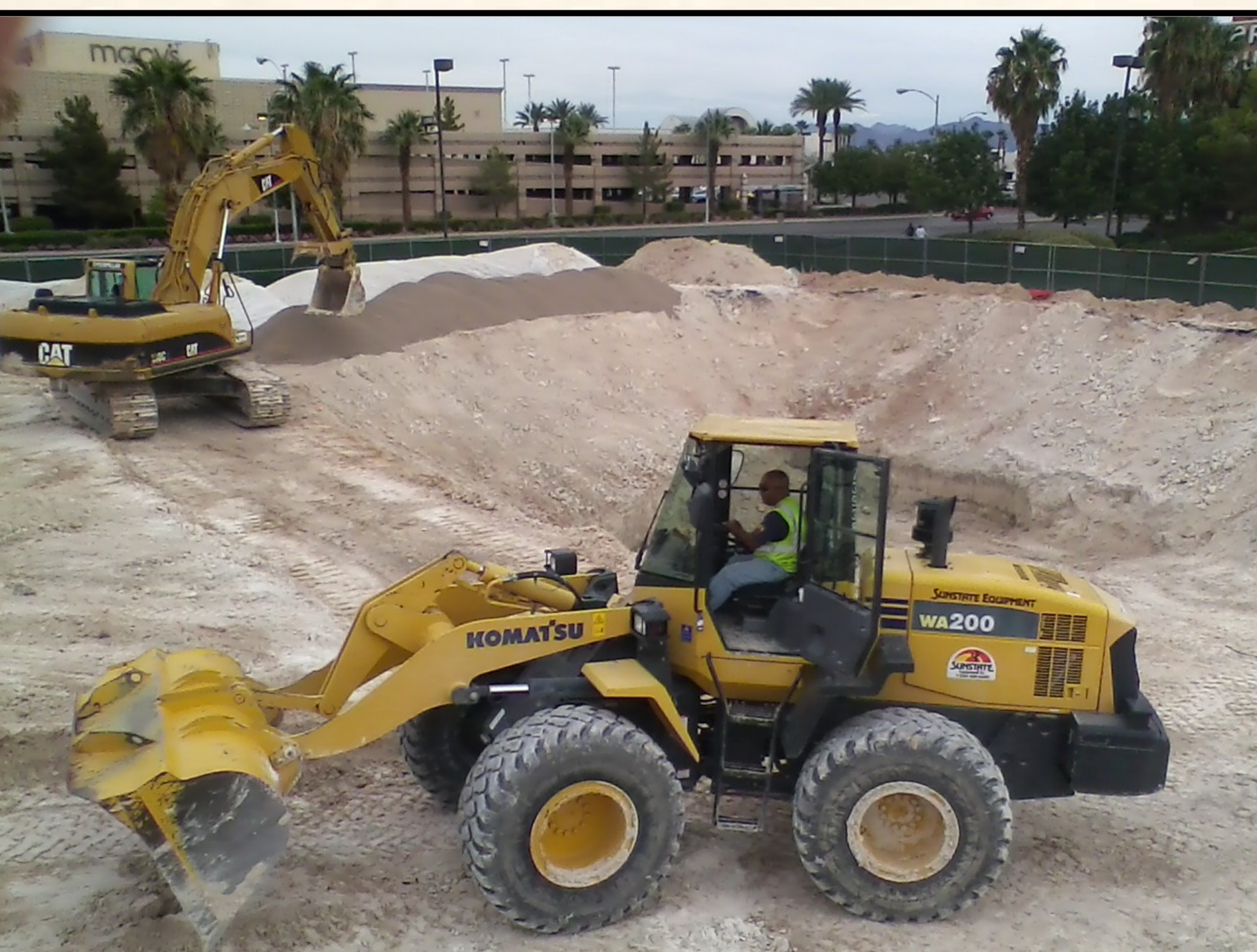
Backfilling after Excavation of PCE Contaminated Soil
