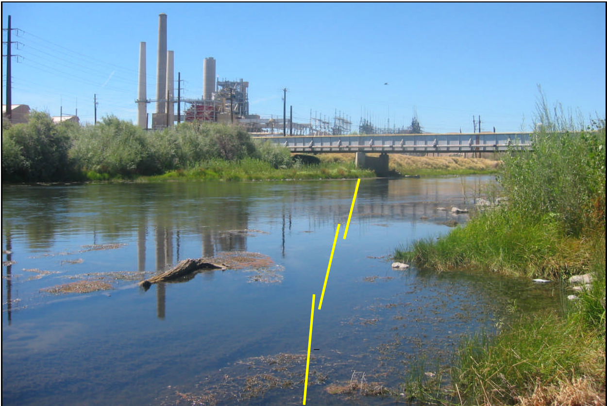
Truckee River Site 12: Tracy Clark Power Station (looking upstream from the north bank)
