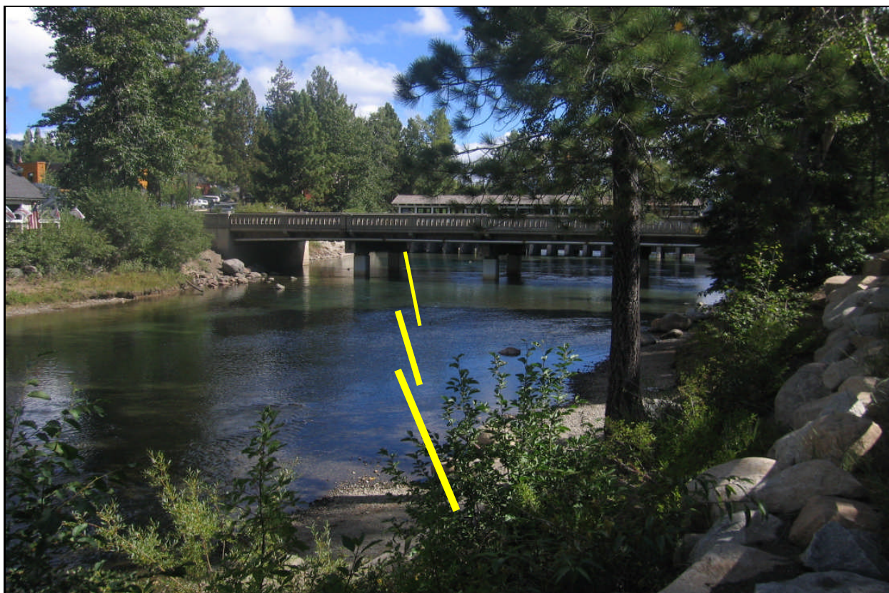
Truckee River Site 1B: Lake Tahoe Outlet Dam – Low Water Conditions (looking upstream from south bank)
