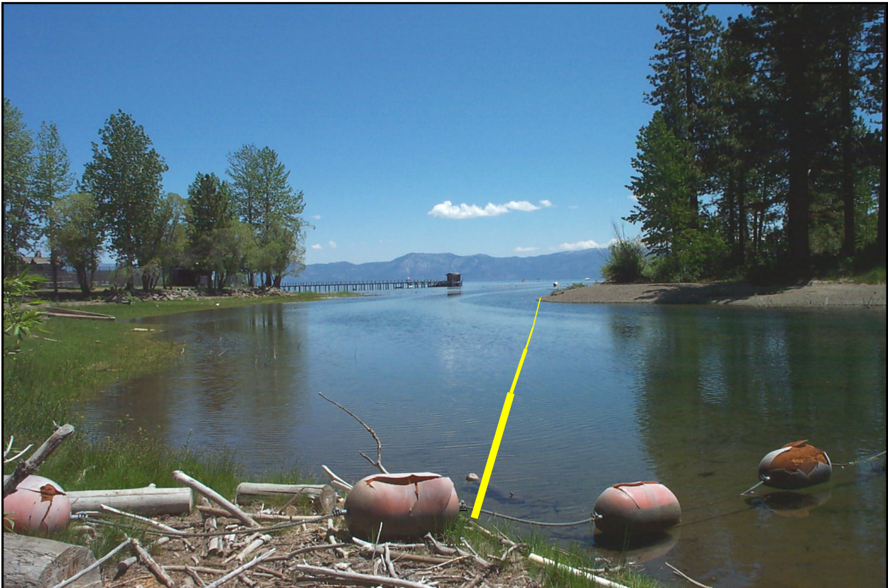
Truckee River Site 1A: Lake Tahoe Outlet Dam - High Water Conditions (looking east from south side of dam)
