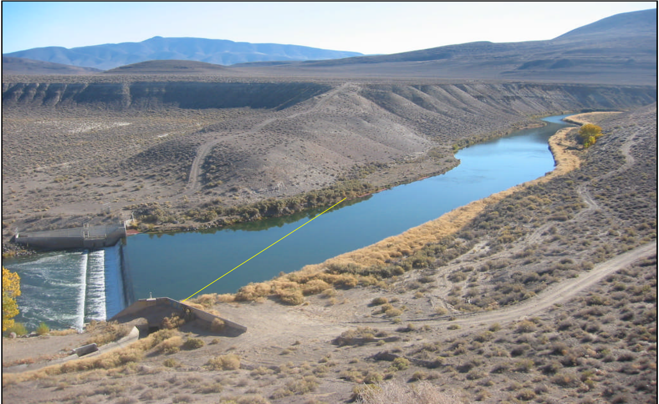
Truckee River Site 17: Numana Dam (looking upstream from the south bank)
