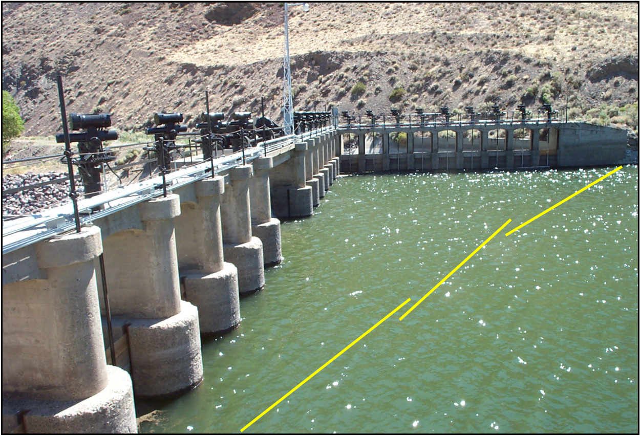
Truckee River Site 14A: Derby Dam (looking upstream from the north bank)
