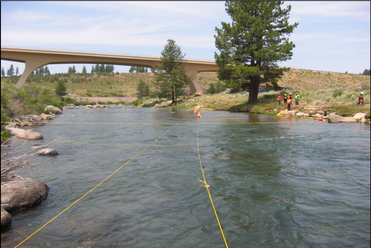
Truckee River Site 6: Glenshire Bridge (looking downstream from north bank)
