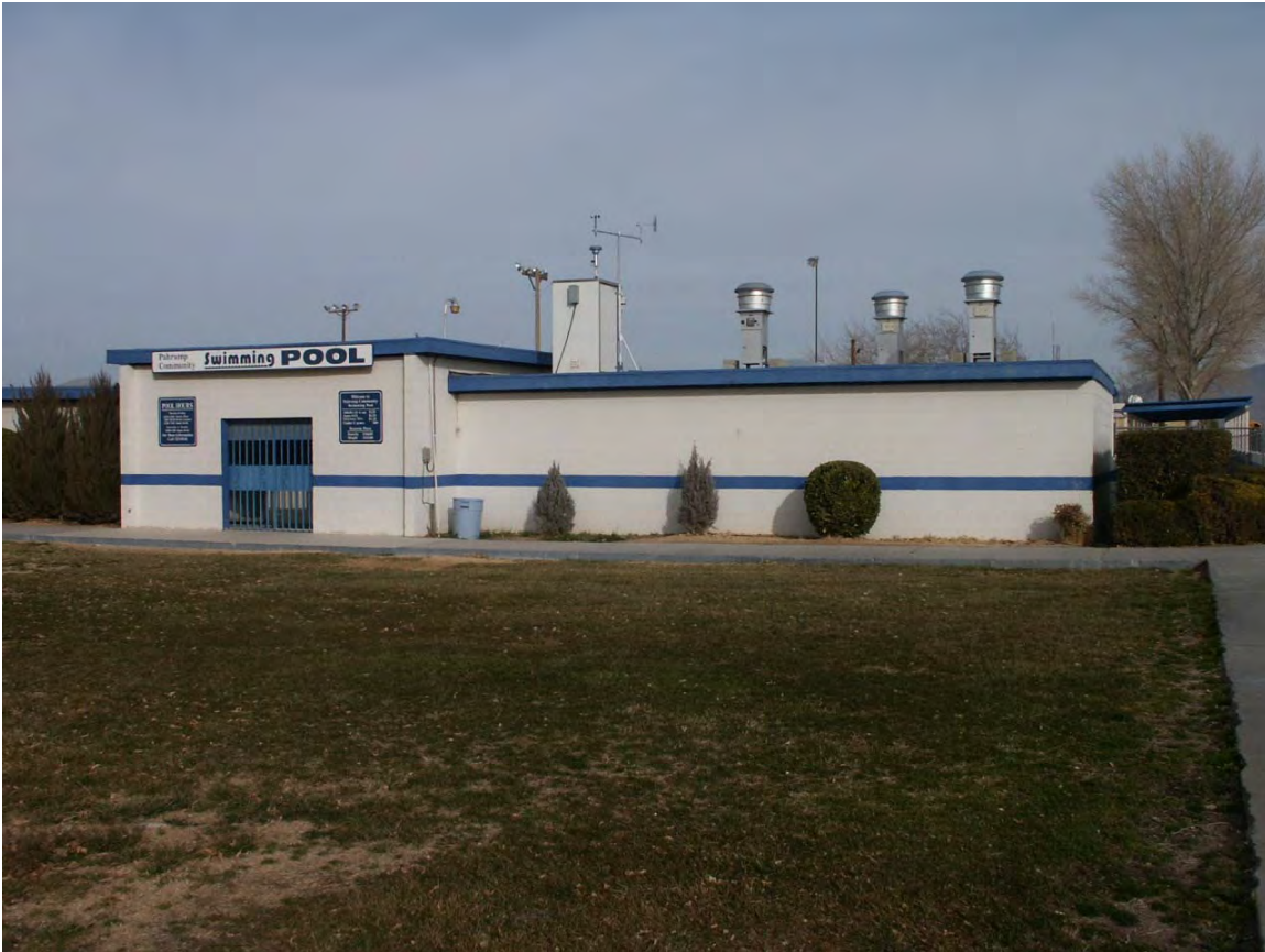
Figure 1. Municipal Pool Monitor. This site has been operational since 2001. Nearby land use is predominately recreational and includes irrigated parkland, rodeo ring, and paved parking lots. Additionally, the county offices and State Highway 160 are within ¼ mile. There are no trees or buildings close enough to affect siting criteria, and the monitor has a 360° unrestricted airflow.
