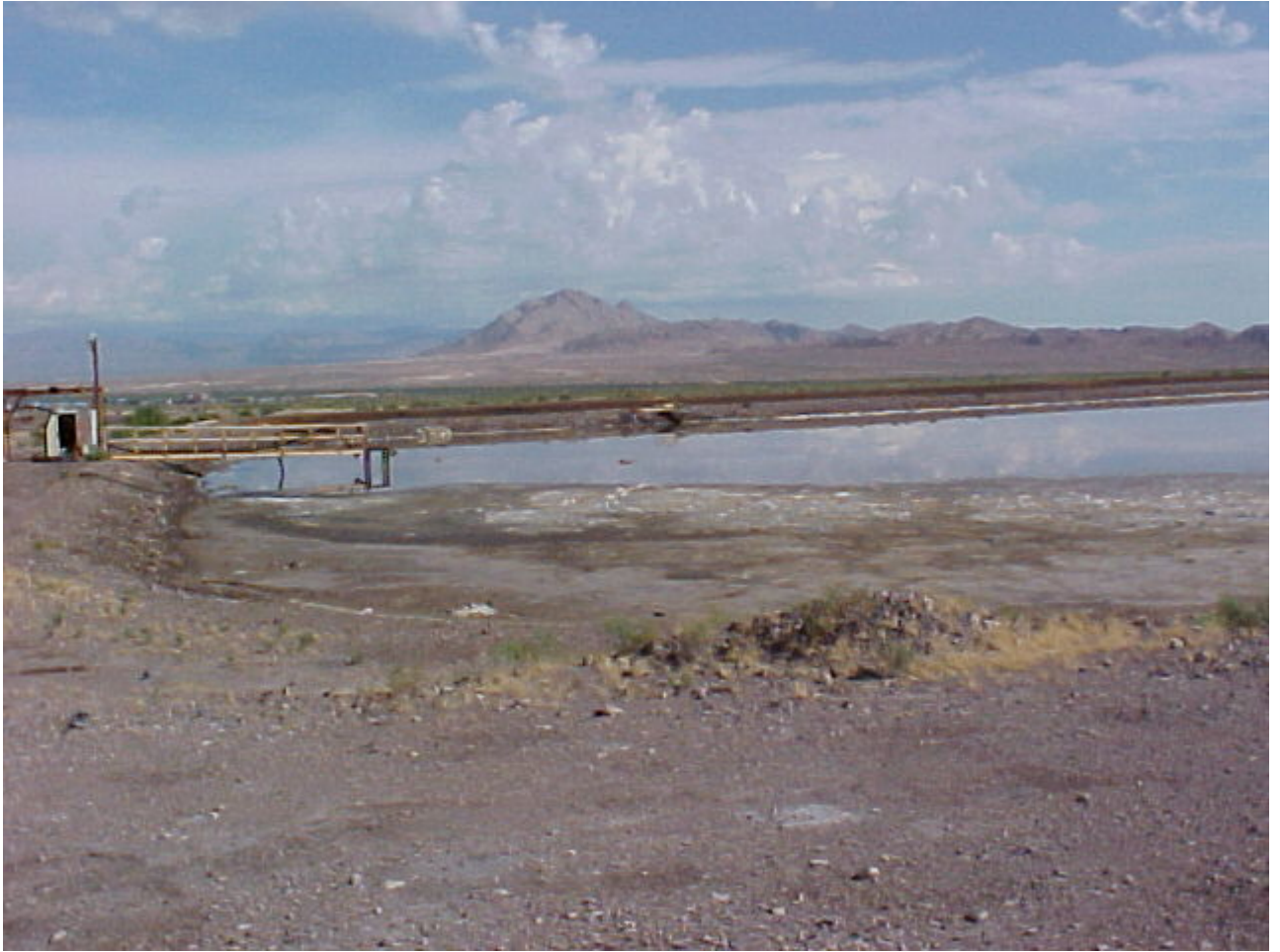
Former TIMET pond located in the Upper Ponds portion of the Site
