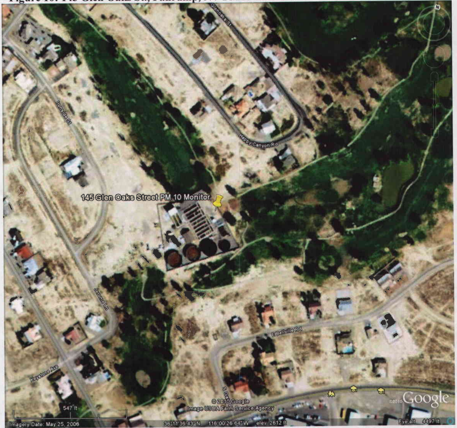
Figure 10: 145 Glen Oaks St., Pahrump, NV PM10 Monitor
